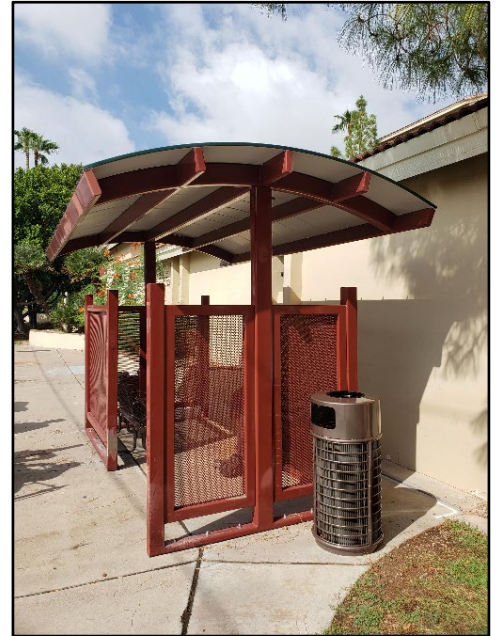
Scottsdale standard bus shelter and associated amenities
