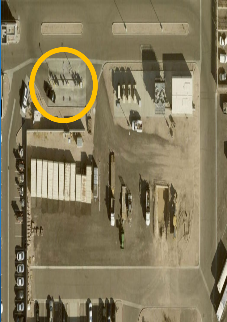
South Corp Yard Diesel Fueling
