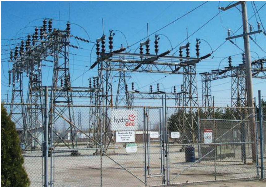
Fence gate is in the normally closed position in this photo.
