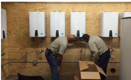
Facilities Staff Install New Point of Use Hot Water System
