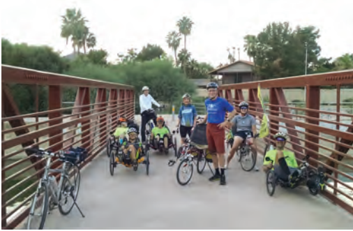
Jackrabbit Bridge on Arizona Canal Path
