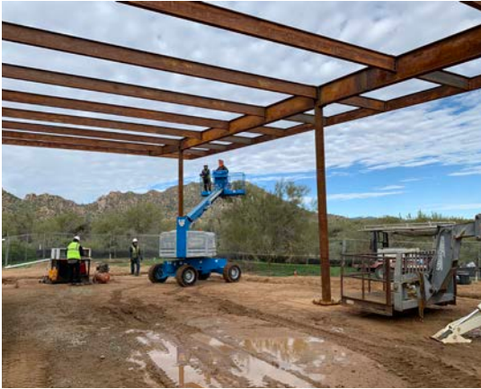
Granite Mountain Trailhead construction
