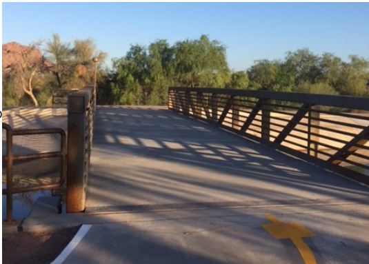
Crosscut Canal Bridge
