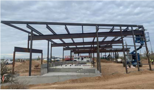
Construction at Pima & Dynamite Trailhead
