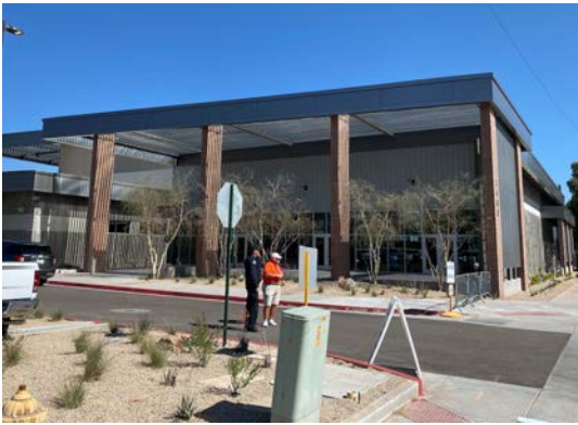
Completed Scottsdale Stadium Renovations
