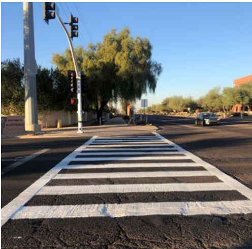
High-visibility crosswalk along Pima Path
