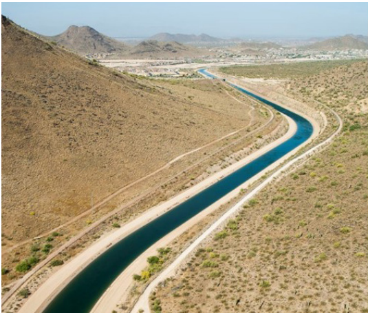
Central Arizona Project Canal running through North Scottsdale
