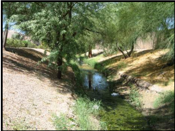
Channel behind Belle Rive apartments
