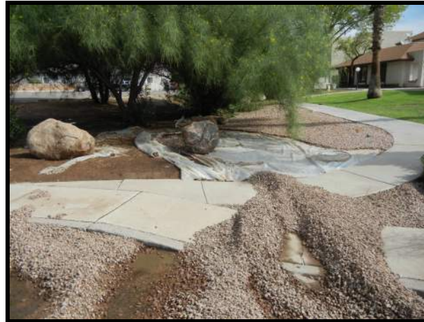
Figure 4-1 Non-structural Property Damage
