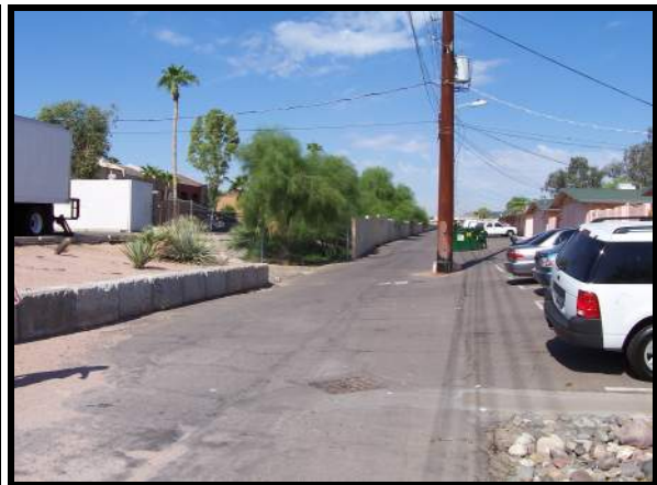
Break in wall for incoming channel flow
