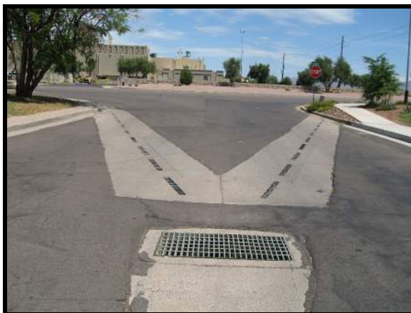
Intersection of Thomas Rd & 87 th St
