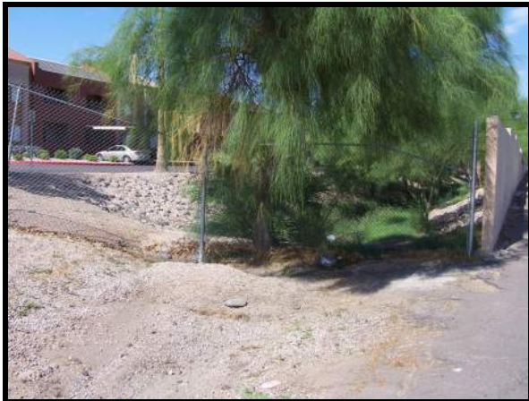
Beginning of channel section
