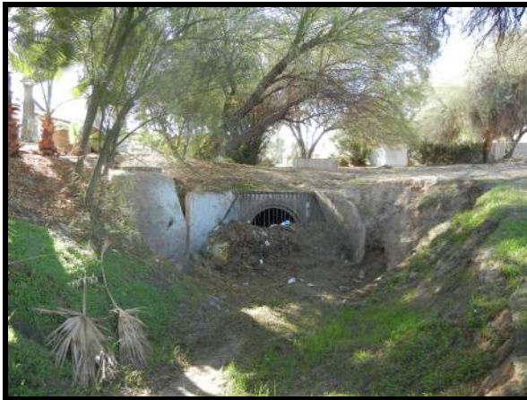
Storm drain entrance at 84 th Pl
