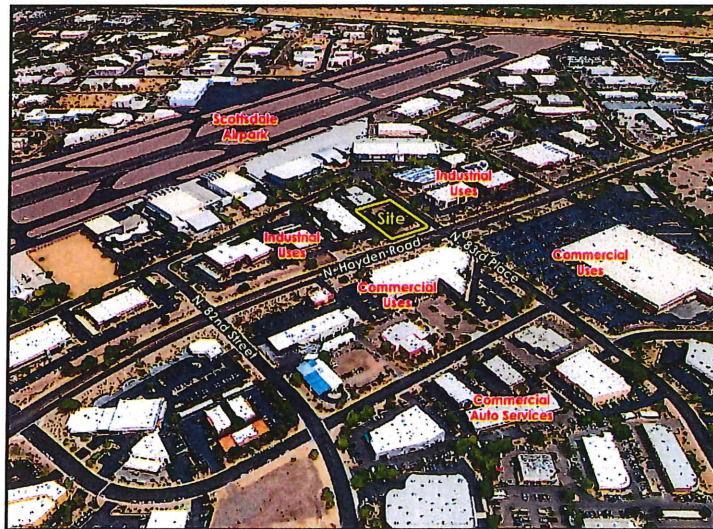
OBLIQUE CONTEXT AERIAL
