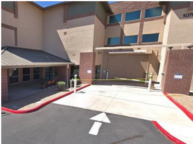
Encourage loading areas in enclosed spaces
