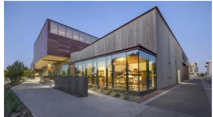
Museum of the West – LEED Gold
