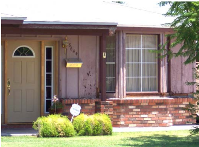
Moving the entrance and adding narrow windows next to the door (multipane sidelights) is not appropriate.
