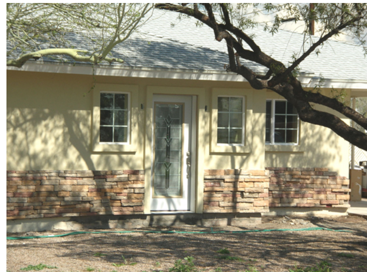
Changing the entry location and replacing the entire door assembly are both strongly discouraged.
