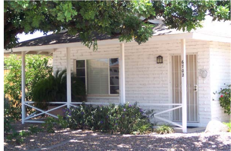
All of the original features of this porch on the L-end of a Village Grove home appear to have been maintained – the modified hip roof, the square wooden posts, and the western style railings.
