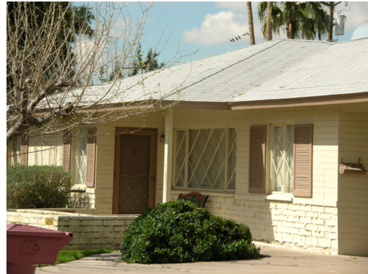
Many homes have the entry door on the side of the L-end of the home. A small porch with one wooden post covers the paved entry patio on this home.
