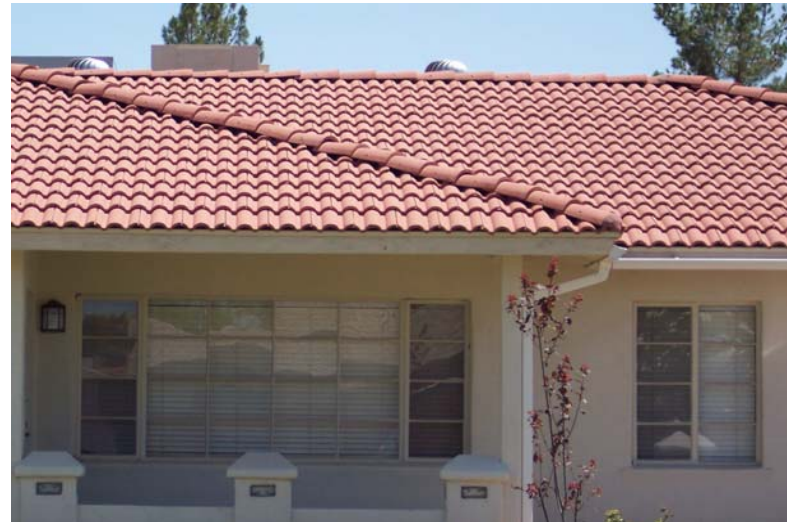
Allied did not use tile roofs in Village Grove. Worn shingle roofs should not be replaced with tile roofs.
