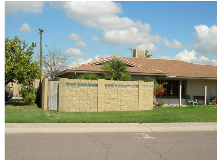
Tall fencing between the street and the front façade disrupts the historic streetscape.
