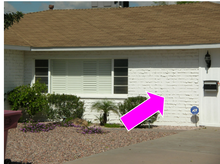
Allied used weeping mortar on their Simple Ranch style homes to enhance their appearance.
