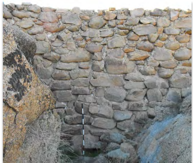
FIGURE 13. HISTORIC ROCK WALL.
