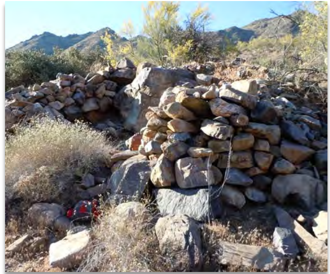
FIGURE 11. UNRECORDED HISTORIC STRUCTURE.
