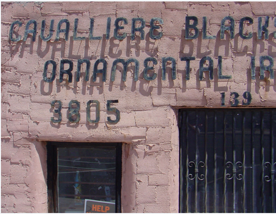
This sign features hand-crafted, torch-cut letters, mounted above a stucco-finished adobe wall - an appropriate sign for a historic blacksmith shop.
