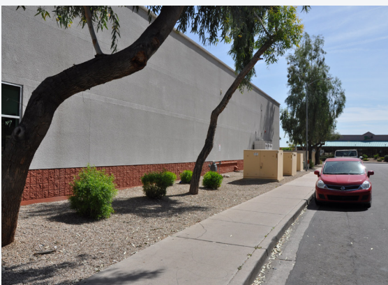
Unscreened electrical equipment and blank building wall is highly discouraged, particularly facing a public street.
