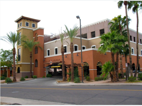
Minimize the apparent mass of a parking structure through building design and architectural features, setbacks, and building articulation.
