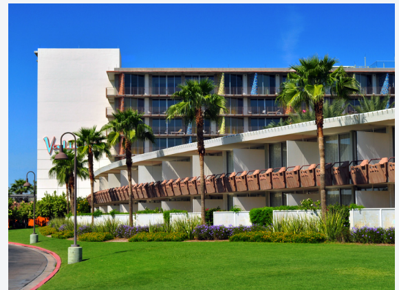
The redevelopment of the Hotel Valley Ho includes the integration of a new tower adjacent to the existing historic hotel (foreground).
