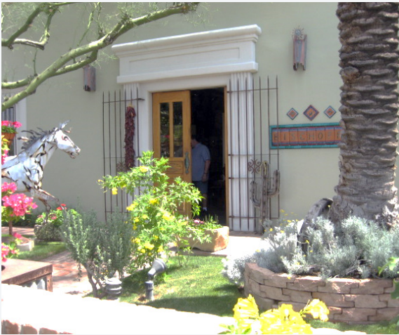
ENCOURAGED - Decorative iron work that enhances the building character while introducing an element of security.
