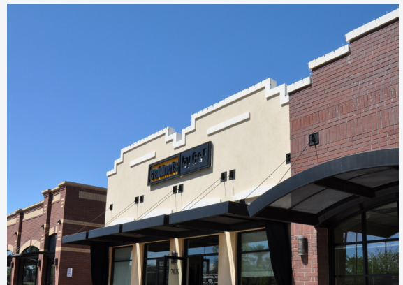
Similar roof forms help to align separate storefronts.
