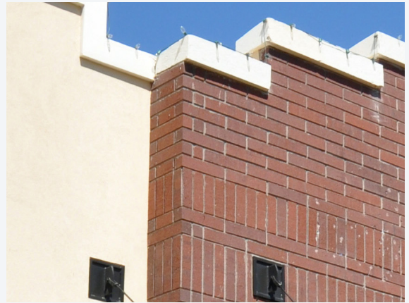
ENCOURAGED - Change in material and color occur with a change in horizontal wall plane.
