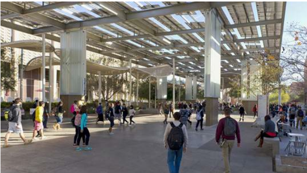
Pedestrian solar PV shade canopy.
