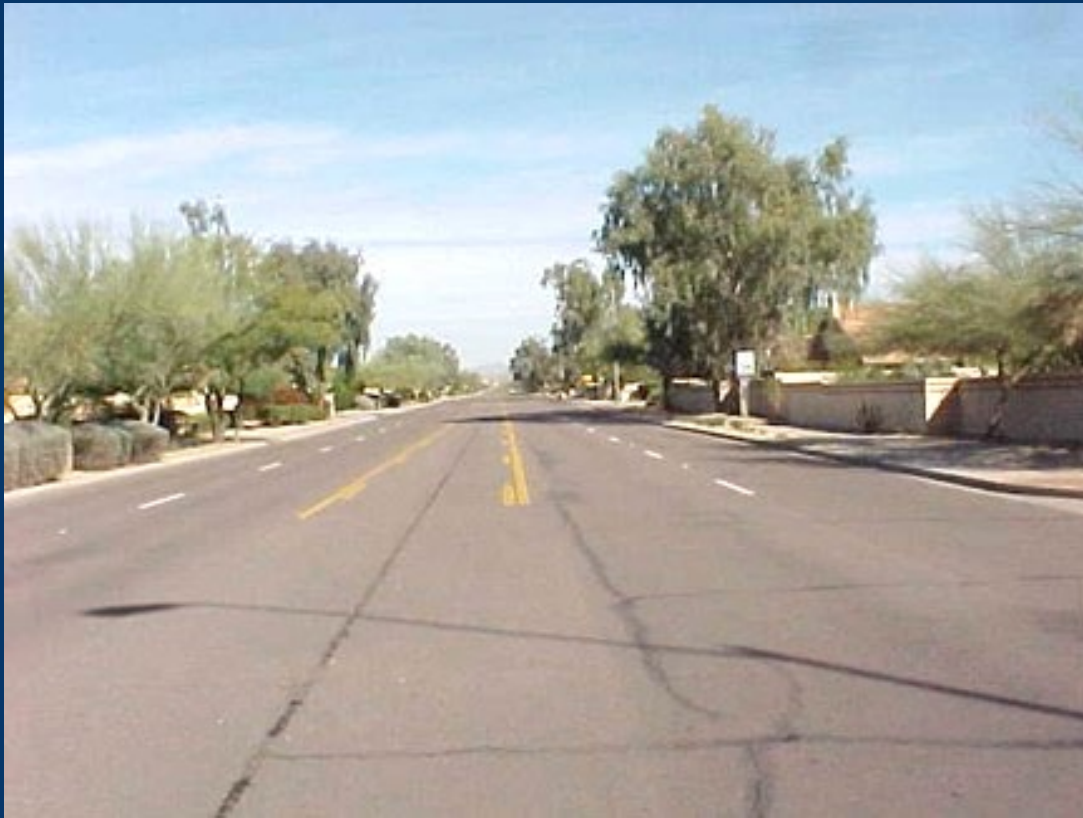
Major Collector 96 th Street - Before
