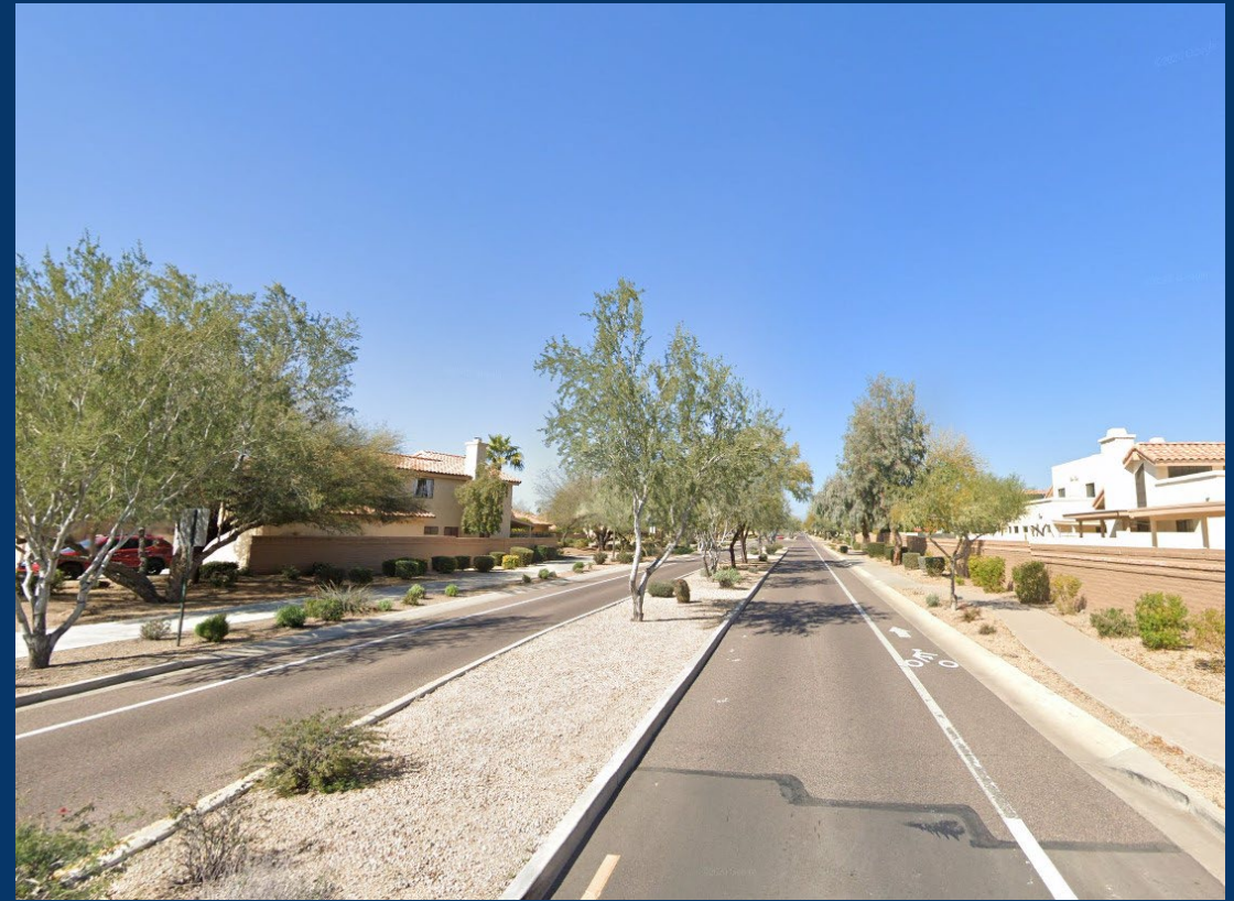
Minor Collector 96 th Street - After
