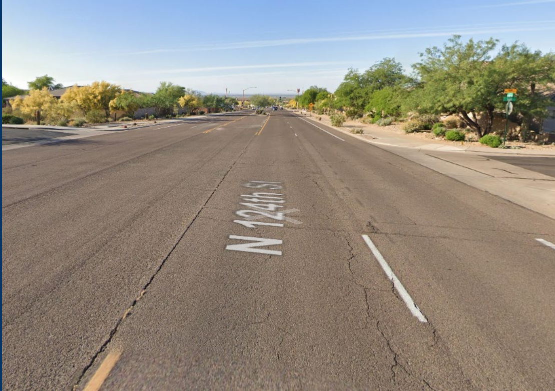
Major Collector 124 th Street - Before
