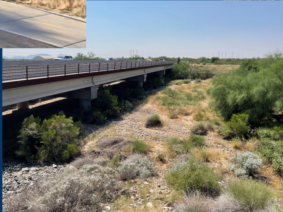
3. Looking west, on north side of existing Bell Road Bridge
