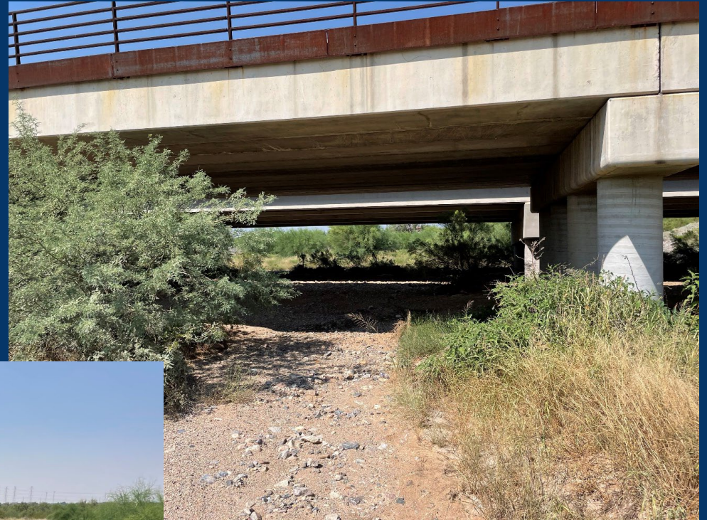
2. Looking north underneath existing Bell Road Bridge
