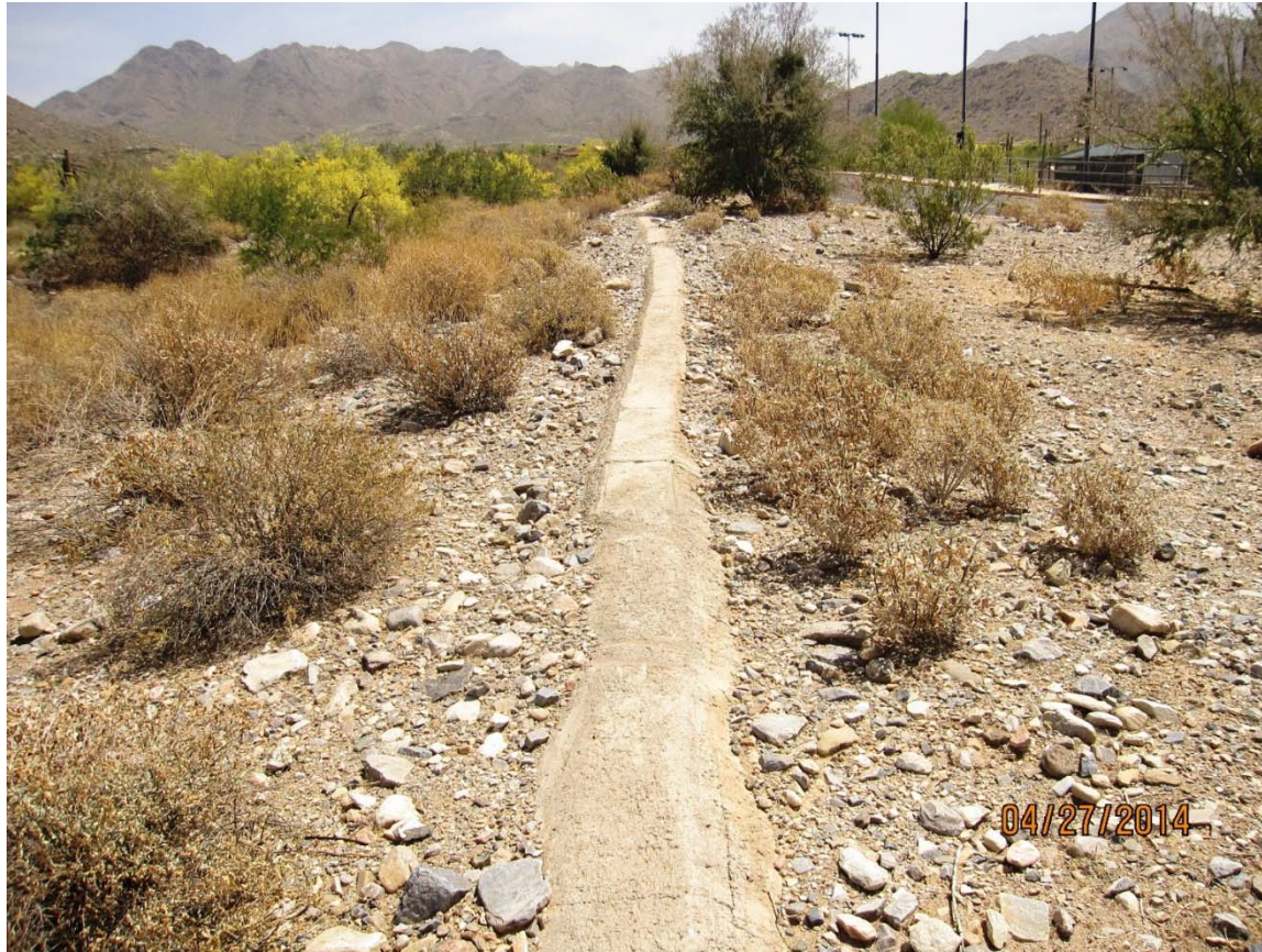
Buried bank protection South of Thompson Peak Parkway – east bank
