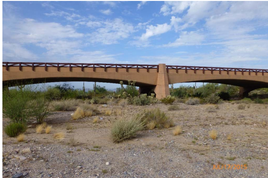
Thompson Peak Parkway bridge
