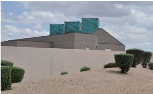
North Indian Bend Wash Granular Activated Carbon Treatment Facility
