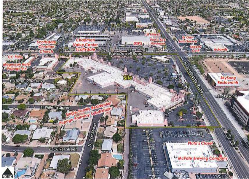
Detail Aerial (facing north)
