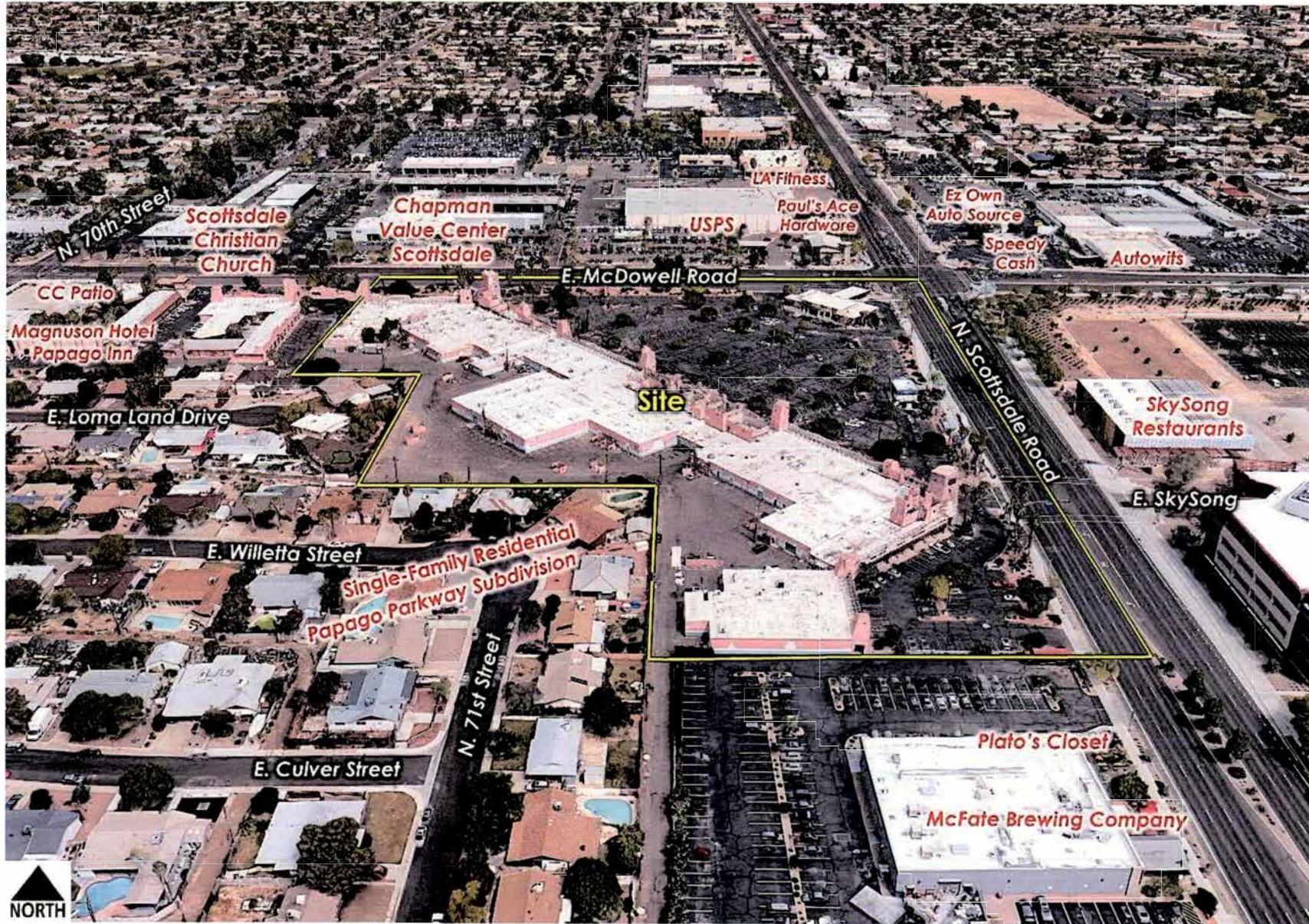
Detail Aerial (facing north)
