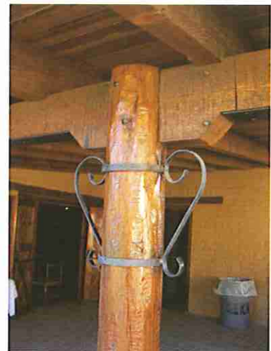
Detail of pealed wooden post, exposed beams and rafters with attached ornamental ironwork.
