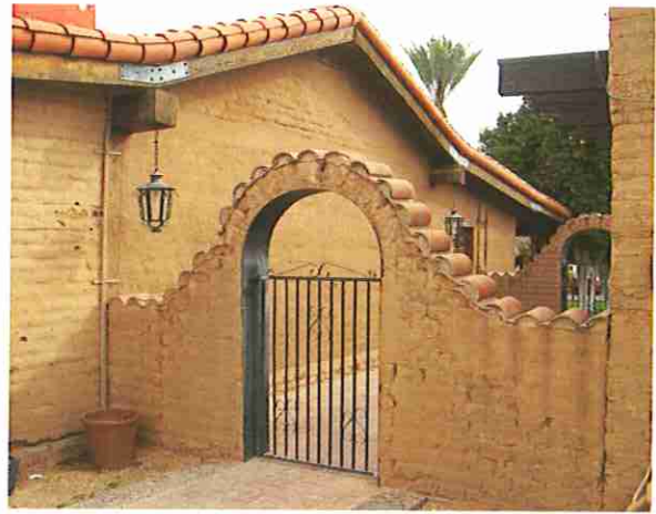
Connecting wall between house and studio.
