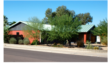
Same house after retrofit
