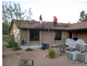
Removing asphalt shingles and replacing them with a standing seam metal roof
