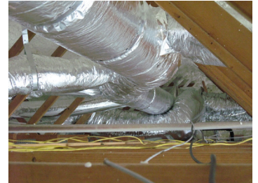
6"-8" Foam insulation to underside of roof surfaces and gable ends plus new HVAC ducts, high-efficiency heat pump and air handler - located on the ground level
