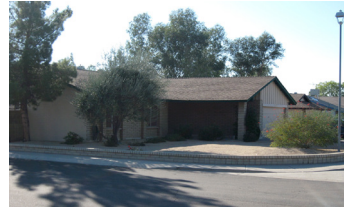
1600sf house before retrofit
