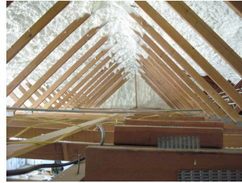
6"-8" Foam insulation to underside of roof surfaces and gable ends plus new HVAC ducts, high-efficiency heat pump and air handler - located on the ground level
