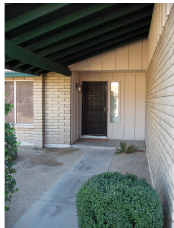
Old front entry. Door set back wasting valuable space. Poorly drained. Subject to puddling in downpours.
