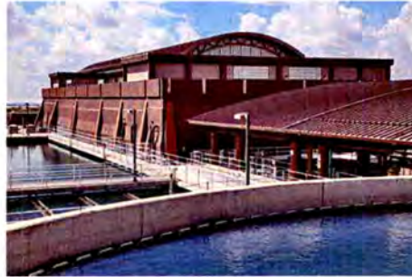
2011 CAP Water Treatment Plant Expansion
