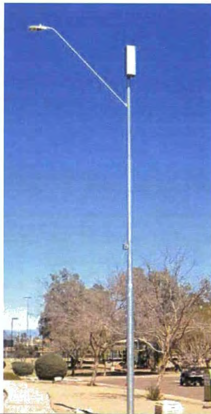
Examples of Built Small Wireless Facilities in Right-of-Way
