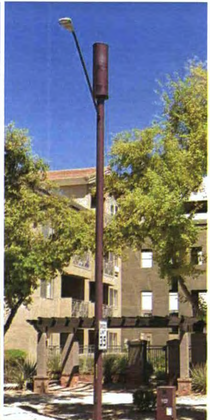
Examples of Built Small Wireless Facilities in Right-of-Way
