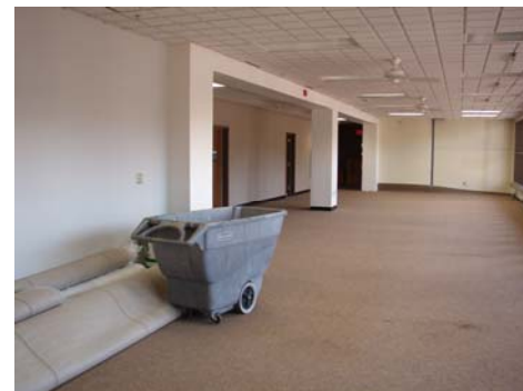
Former Records Unit being converted to office space for Investigative Services
