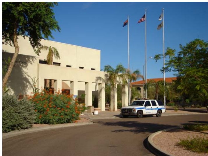
Former Police Headquarters on Via Linda
