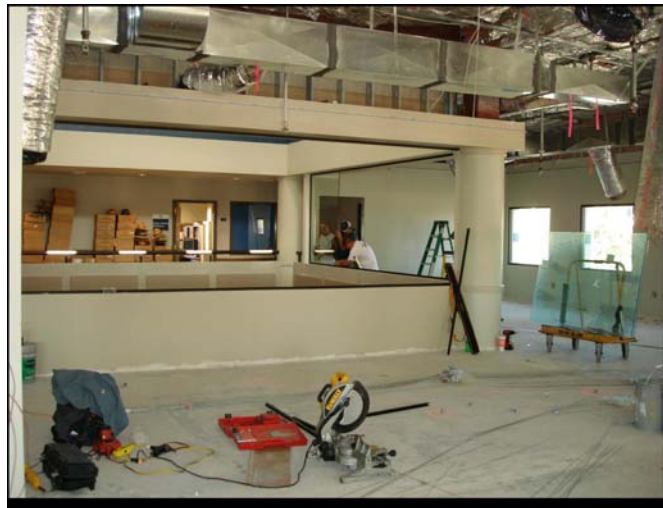
Construction of the new Communications Center
