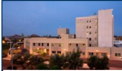
Scottsdale Shea Medical Center trauma center looking east from Piper Place
