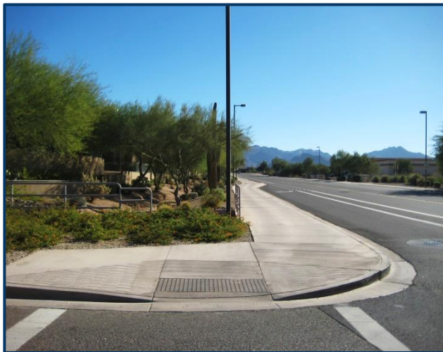
Curb Ramp by Appaloosa Library
