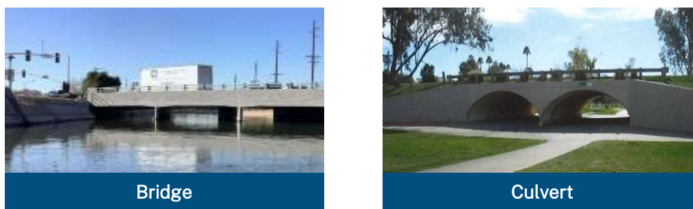
Figure 1. Example of City-owned bridge and culvert.
