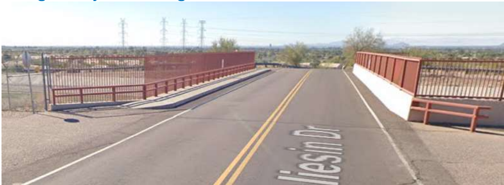
Figure 5. Image of City-owned bridge on Taliesin Drive.
