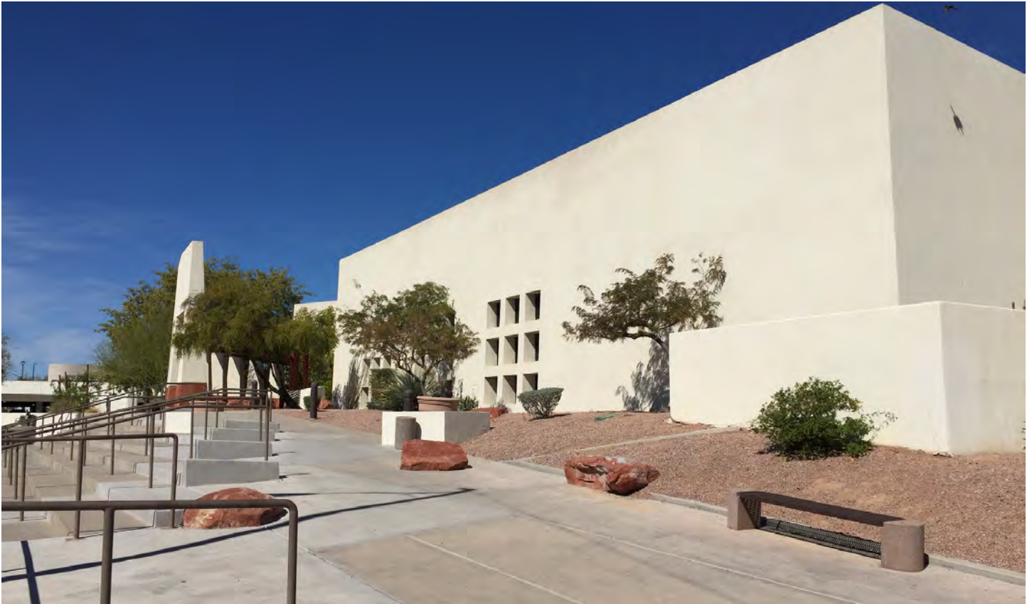
Looking North West
