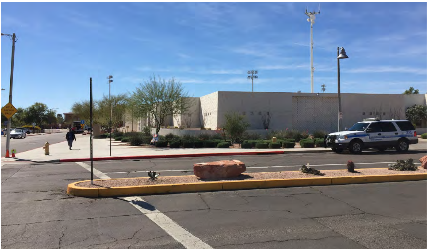
Looking South West
