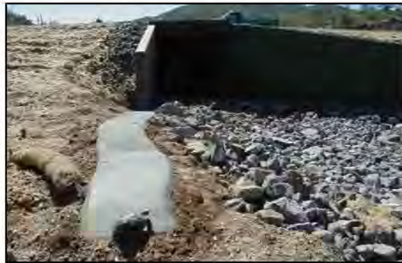
Figure 6. Example Concrete Path for Wildlife Movement Photograph courtesy of Arizona Department of Transportation
