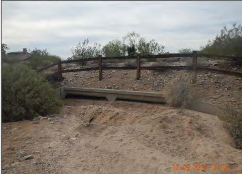
Figure 5-6 Reata Wash North Flood Protection – Openings at Design Approximate Levee Station 21+00
