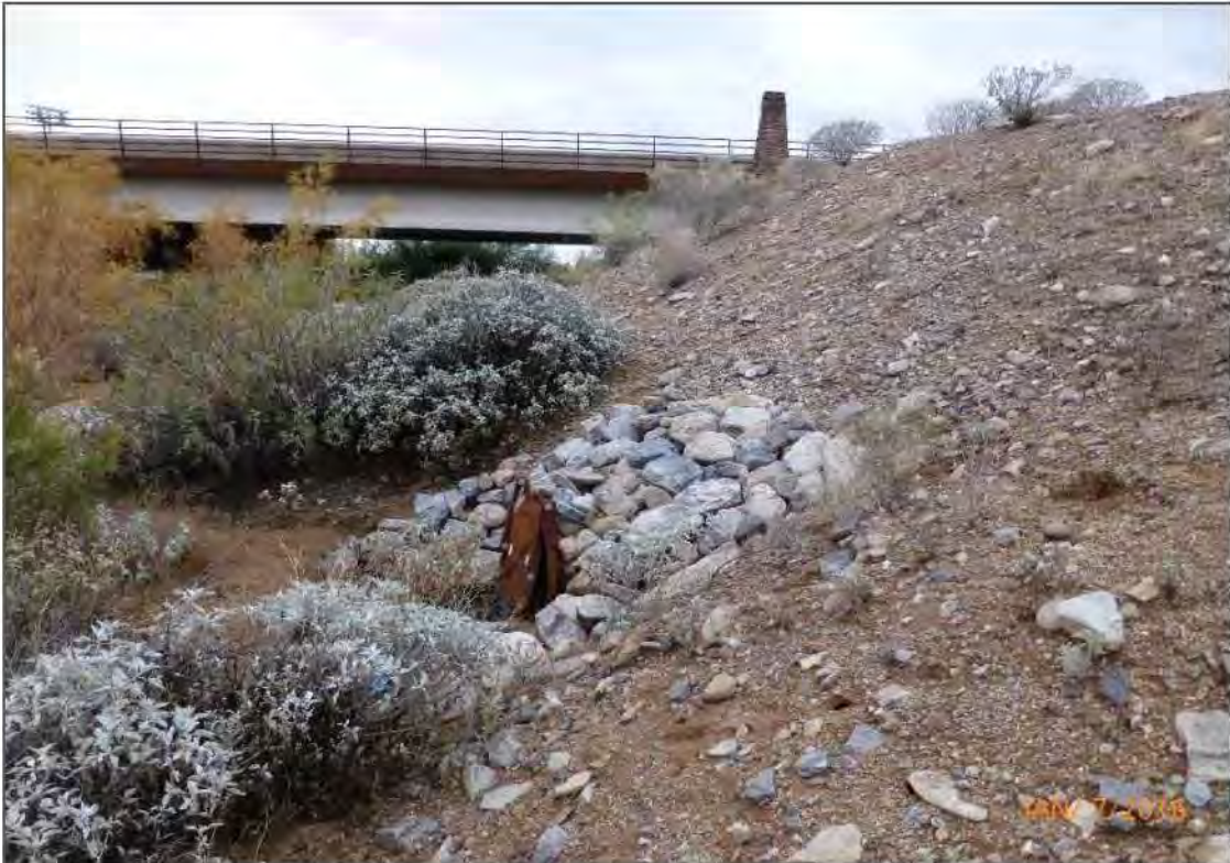
Figure 5-4 Bell Road Levee Flap Gate at Approximate Levee Station 11+00
