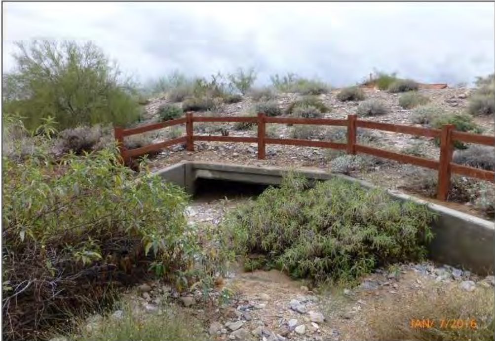
Figure 5-5 Reata Wash South Flood Protection – Openings at Design Approximate Levee Station 21+15
