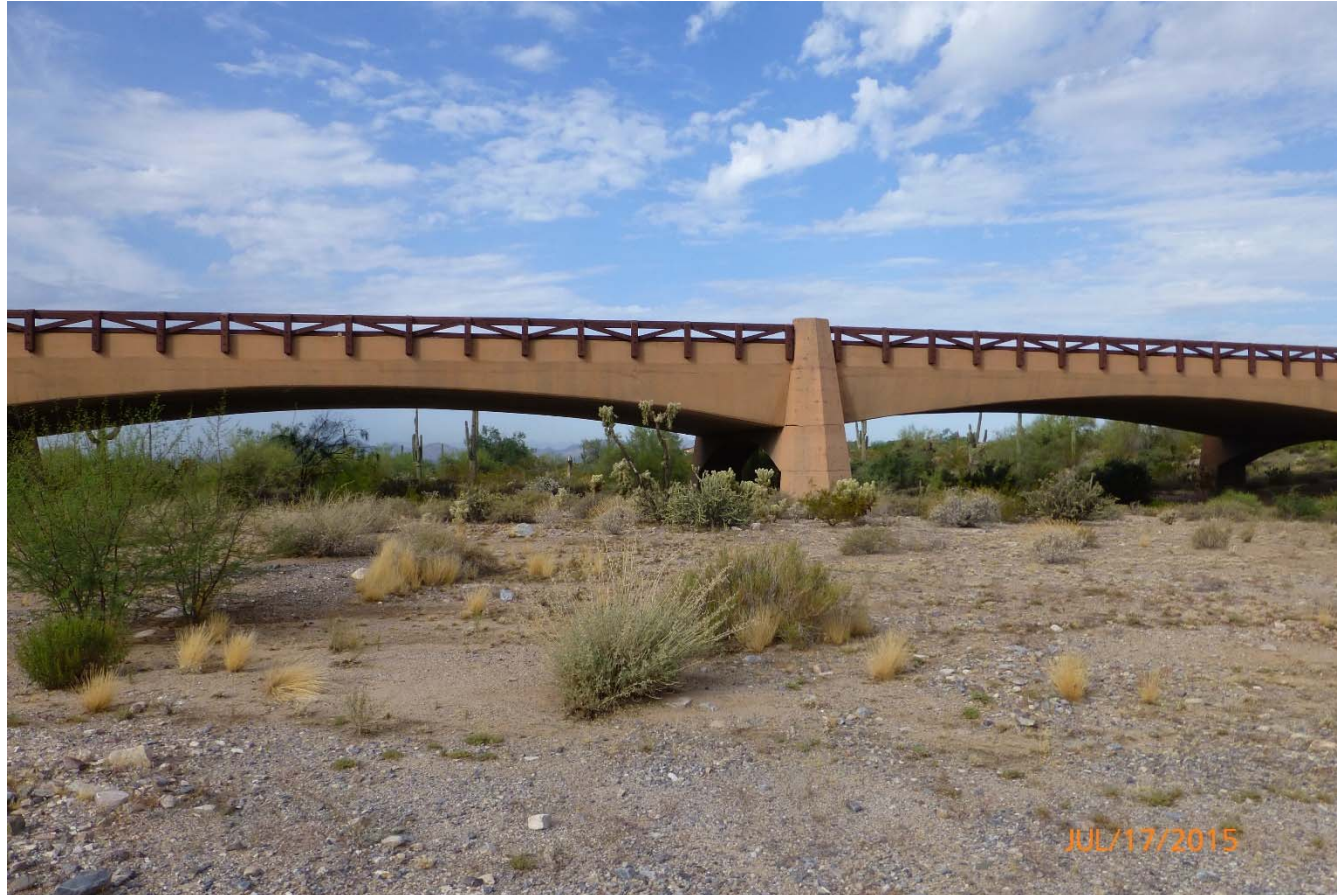
Thompson Peak Parkway bridge
