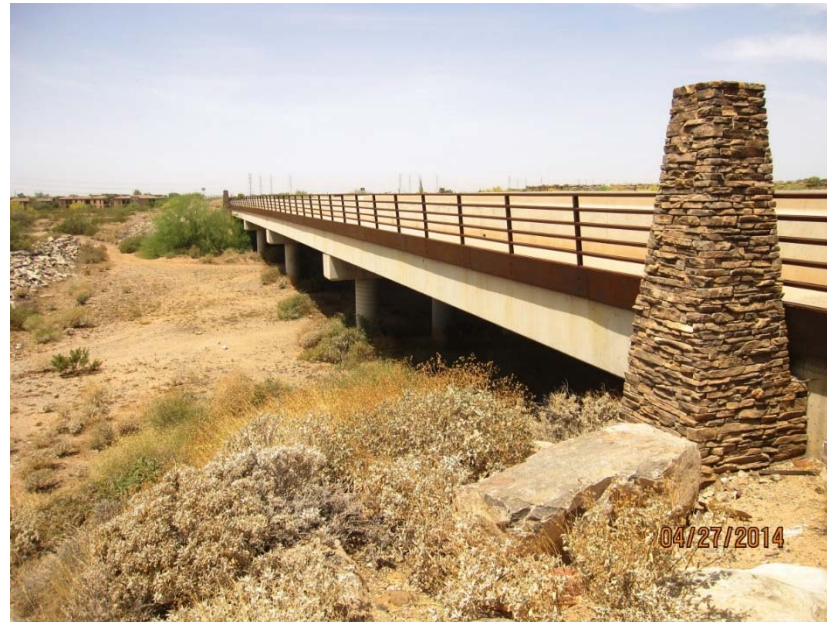
Bell Road Bridge
