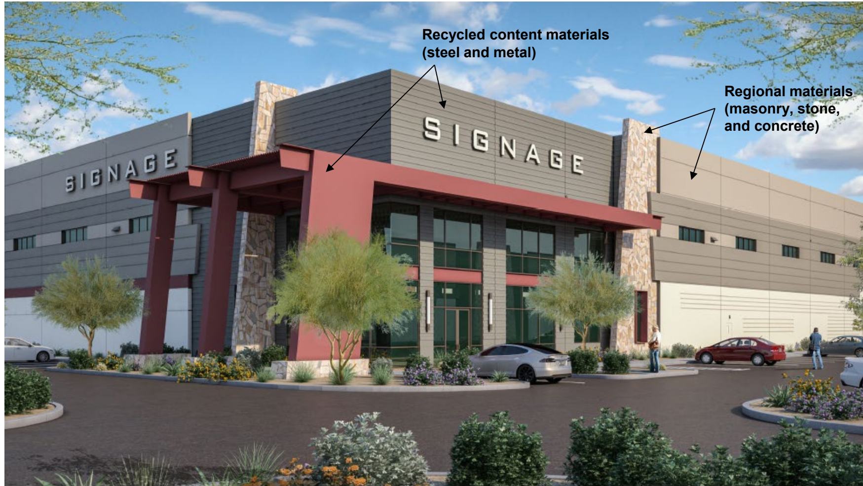
Core and Shell building
