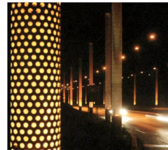
Light pole wraps to match decorative metal panels for Segment 4 (Dry Wash)
