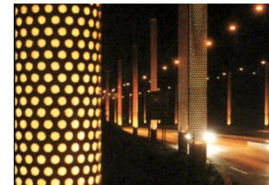
Light pole wraps to match decorative metal panels for the Segment 2 (Homestead)
