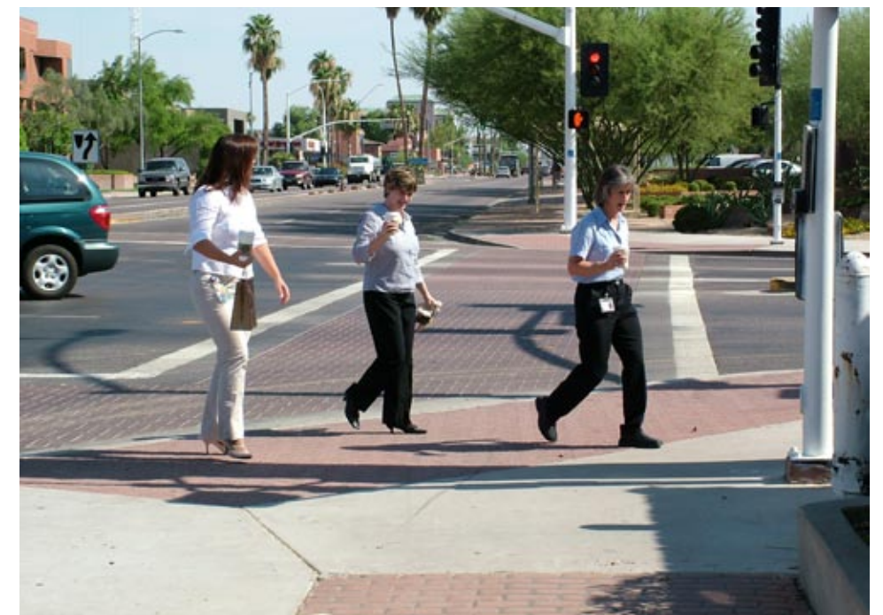
Existing stamped pavement at corners and in crosswalks creates an uneven, heavily textured surface that is difficult to walk on and causes undesirable vibration for wheelchair users.
