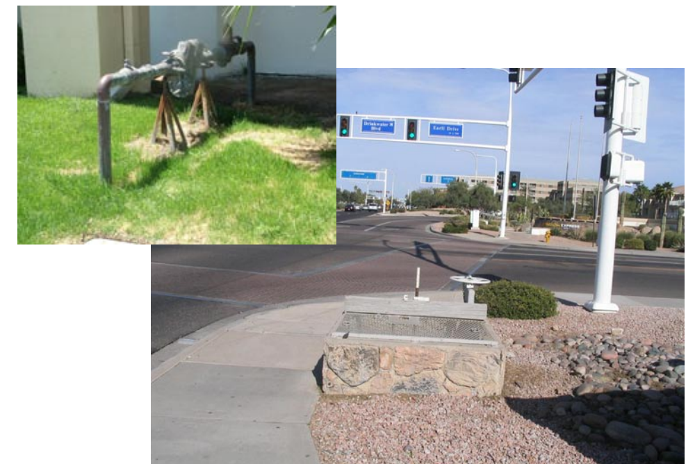
Various utilities and Salt River Project facilities exist within the right-of-way
