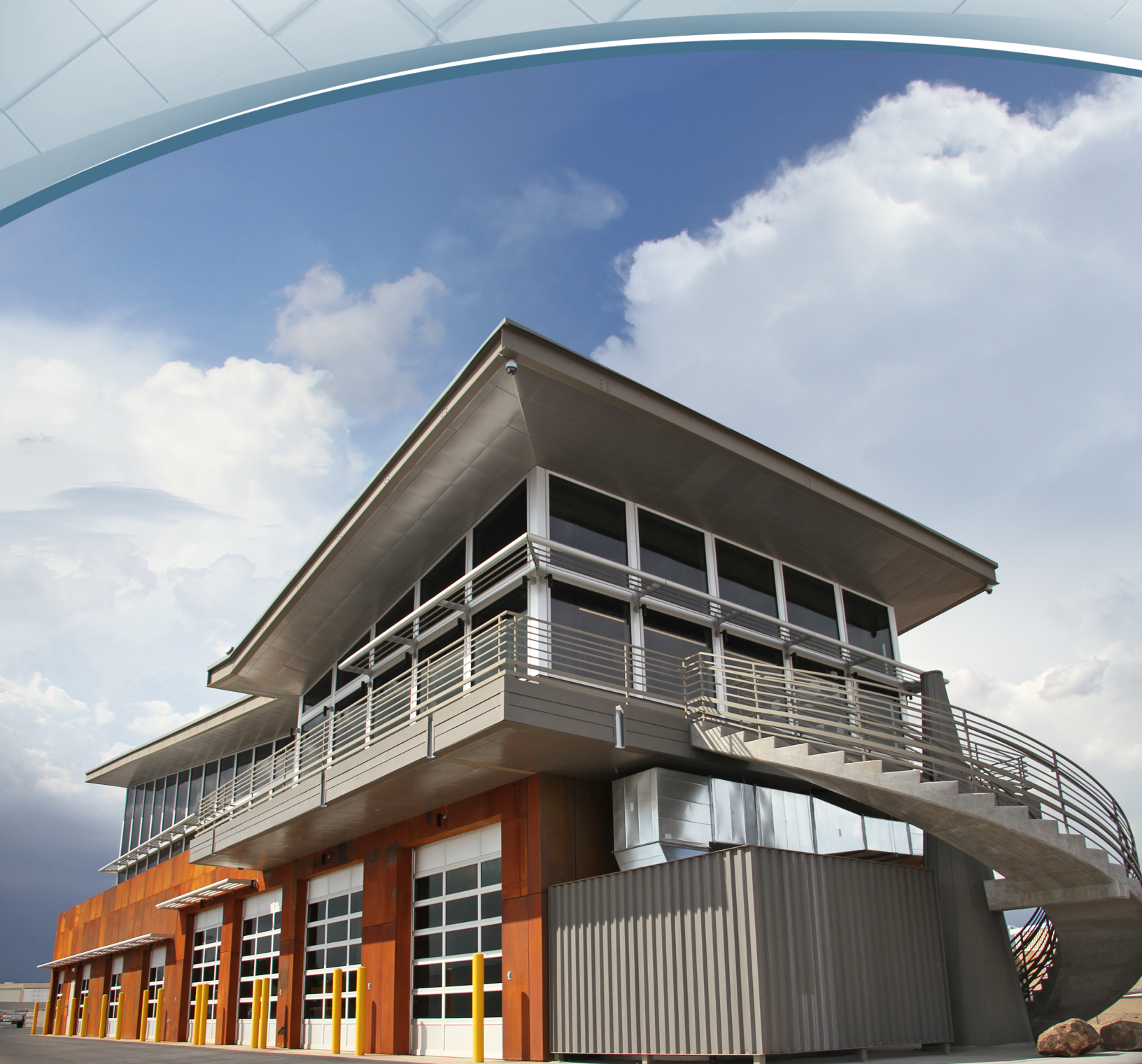
Airport Operations Center
