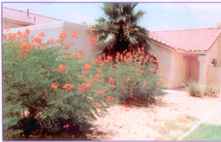
A typical suburban Scottsdale home consisting of lightweight construction and a heavy tile roof. (CS6-1)
