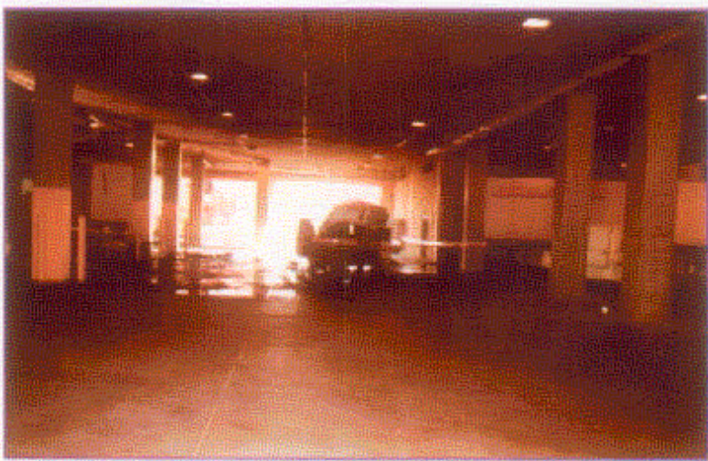
View of the loading dock area and the involved ambulance unit. Five sprinkler heads activated and helped control the fire. (CS 1-5)
