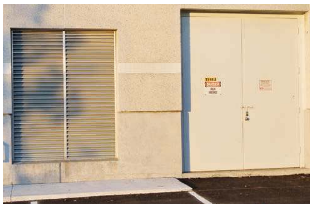
Exterior access transformer vault door and ventilation
