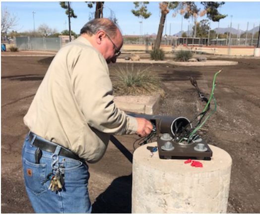
Facilities Staff rewires a park light pole
