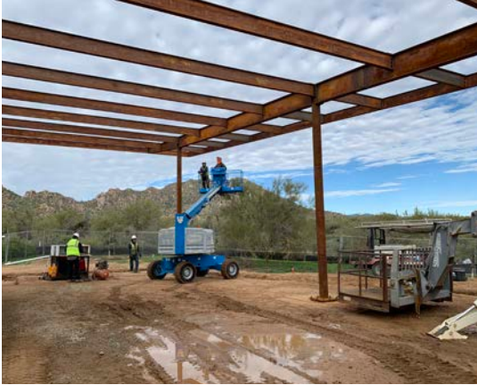
Granite Mountain Trailhead construction
