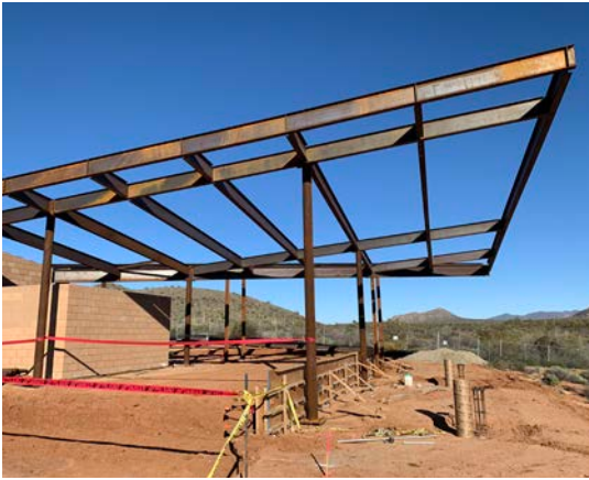
Fraesfield Trailhead construction
