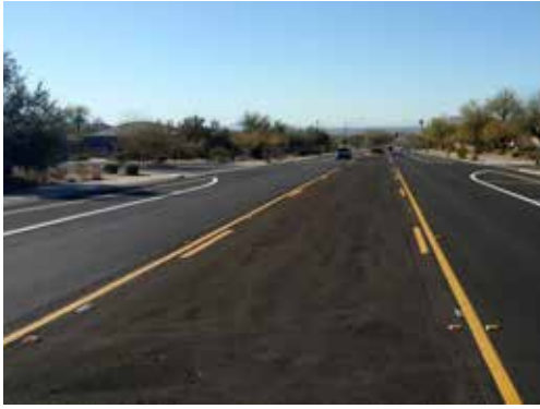
New pavement and striping on 124th Street
