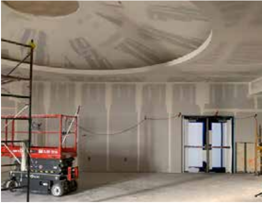
Civic Center storytime room construction
