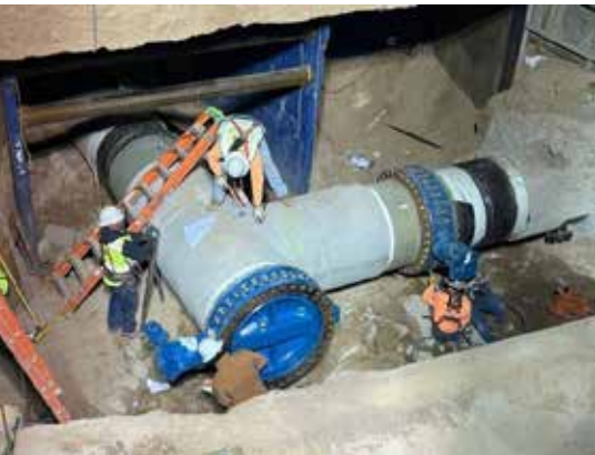
Scottsdale Water maintenance crew work on a main water line
