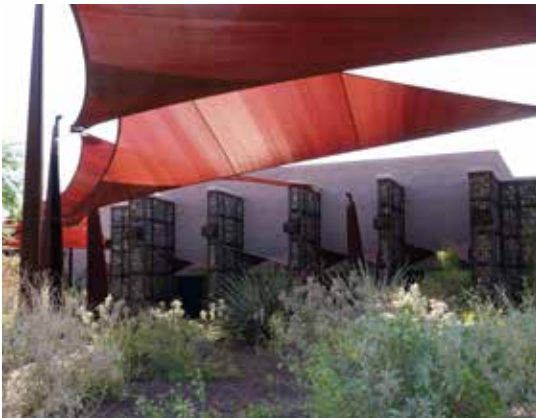
Scottsdale Water operates seven water facilities including Chaparral Water Treatment Plant
