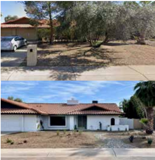
OFI landscape renovation and painting done on a Cactus Corridor residence - Before & After
