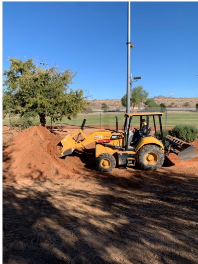
Turf removal at Horizon Park on Scottsdale Road.
