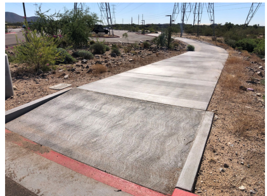
North end of Bell94 Sports Complex Path.
