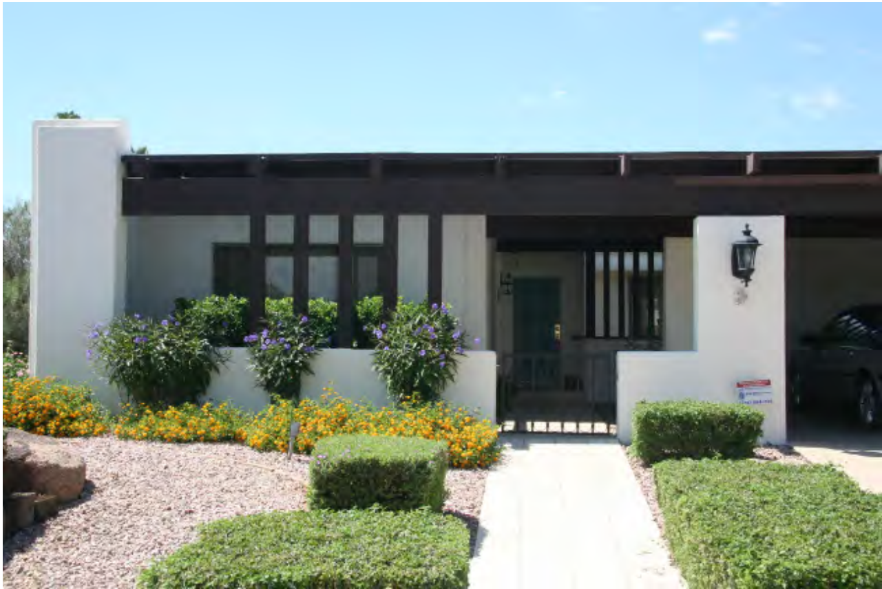
Lot 30, Type A - Low wall with wood post screening and wrought iron gate
