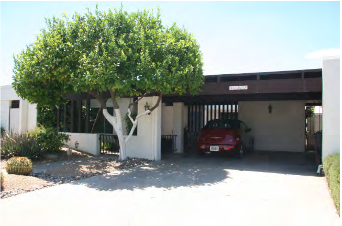
Lot 23, Type A1 - Wood post screen on stucco wall and wrought iron gate
