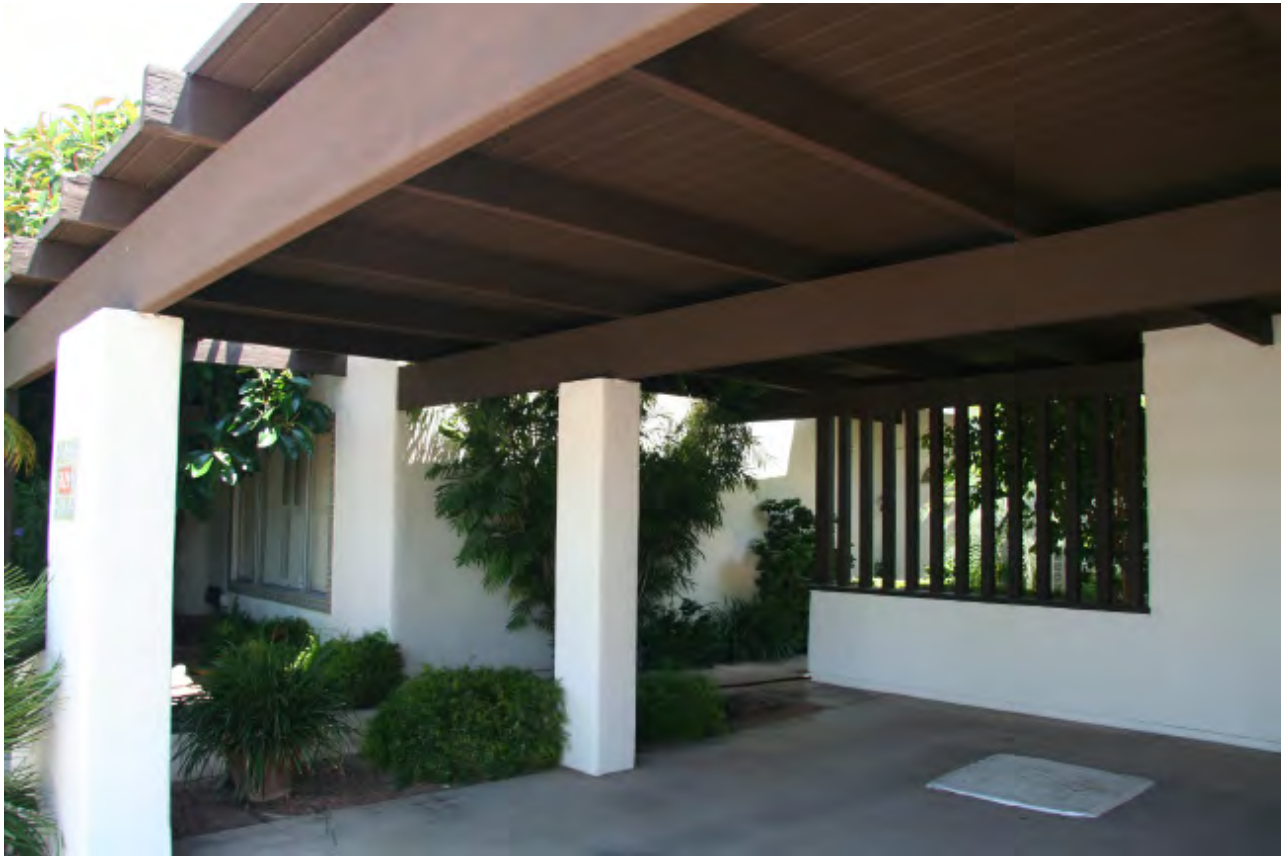
Lot 51, Type A1 - Wood beams and exposed rafters
