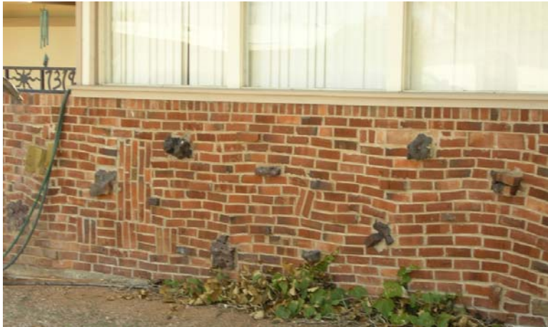
Clinker brick is perhaps the most distinctive and rare feature found in the Town and Country neighborhood.
