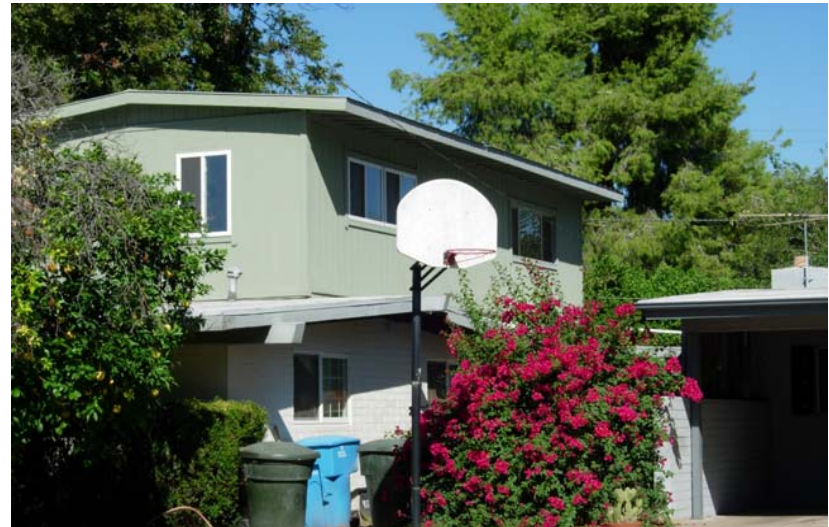
Second story additions on houses with very low pitched roofs, such as Haver houses, accentuate the height being added and are not appropriate.
