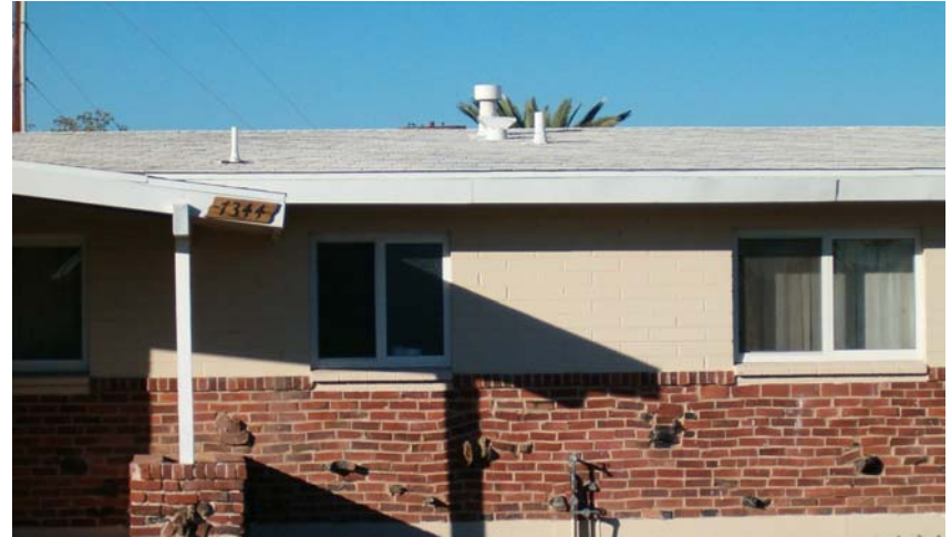
Clinker brick is an extremely rare wall material that actually common in the Town and Country neighborhood. It should be retained and left visible in all cases.
