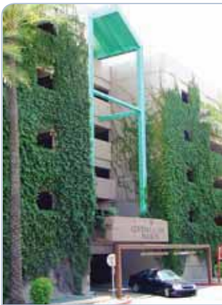
Vines on solid wall surfaces can help cool public spaces where there is little room for shade trees.
