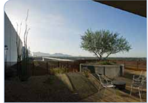
Stormwater retention can sometimes be addressed using green roof technology. Photo source: Henkel.
