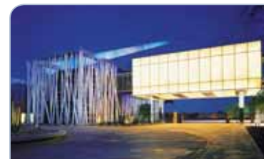
Hangar One celebrates aviation in its architecture by incorporating a representation of a paper airplane into the building. Photo source: Tihany Design.
