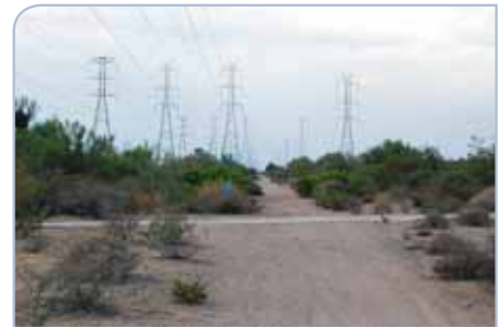
The power line corridor on the northeastern boundary of the Greater Airpark provides electric service to Scottsdale.
