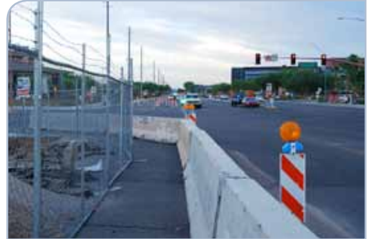
Capital improvements, such as road construction and pipe upgrades, should be coordinated whenever possible.
