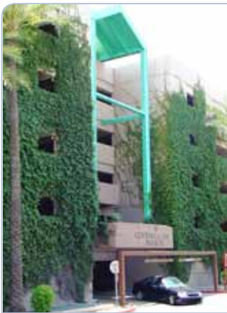
Vines on solid wall surfaces can help cool public spaces where there is little room for shade trees.
