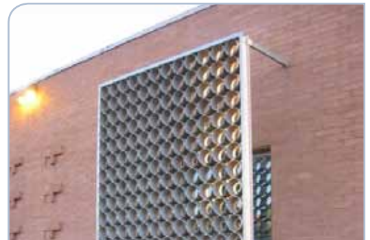
Sun screens can be incorporated into building architecture to reduce heat absorption.
