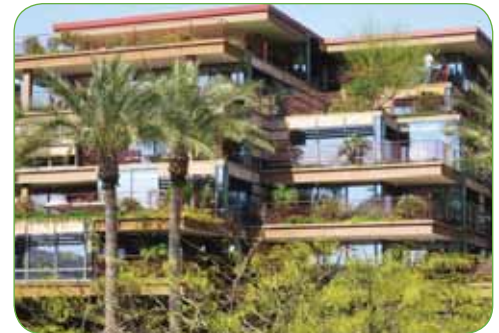
Design responding to unique, Sonoran climate (green roof, recessed windows, etc.).
