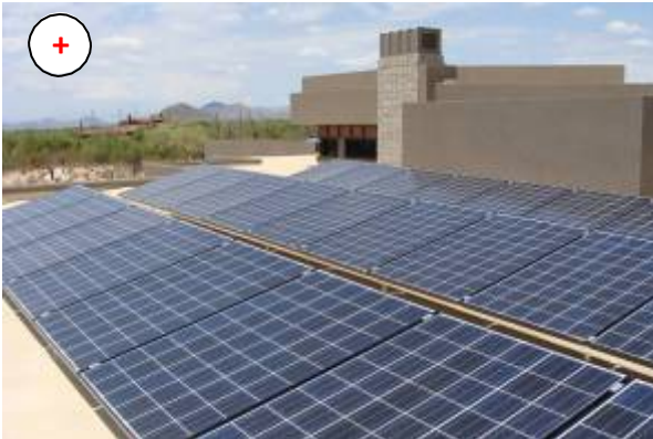
Solar panels on flat roof without parapets.
