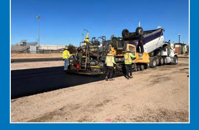
Crews working alongside the paving equipment inspect the surface and shovel and rake material to ensure edges and pavement transitions are smooth. Large vibratory rollers are used to compact the material.
